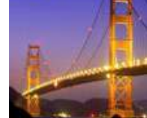
Golden Gate Bridge San Francisco
