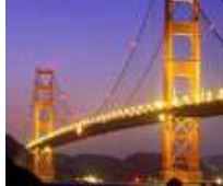
Golden Gate Bridge San Francisco
