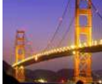
Golden Gate Bridge San Francisco
