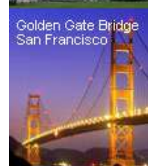
Golden Gate Bridge San Francisco
