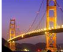
Golden Gate Bridge San Francisco
